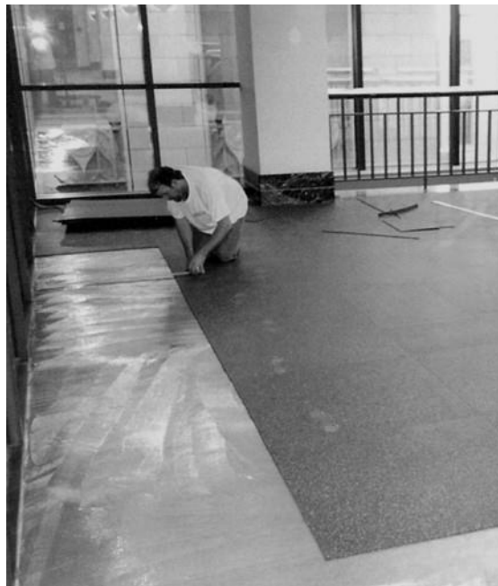
Square Cut / Glue Down Installation
