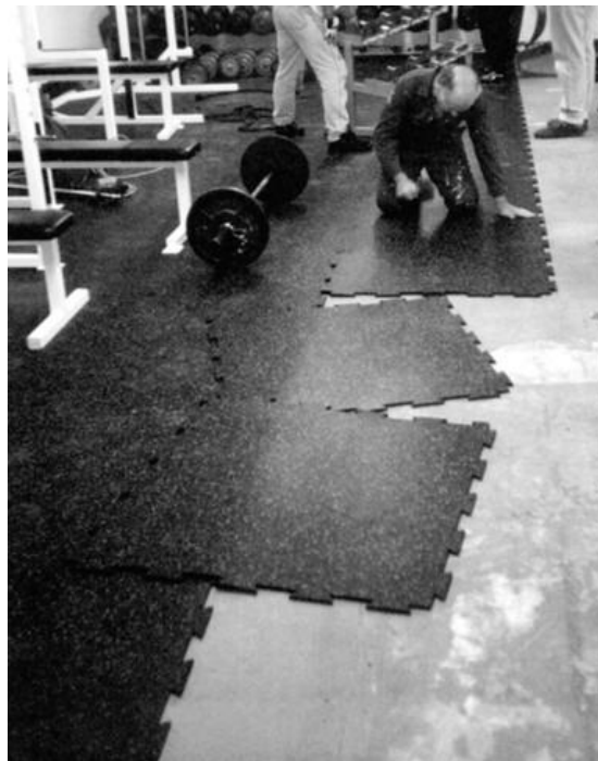
Four-Side Interlock Loose Lay Installation
