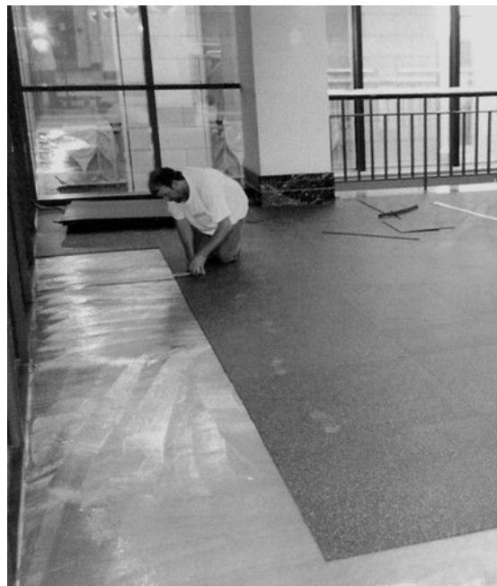
Square Edge / Glue Down Installation
