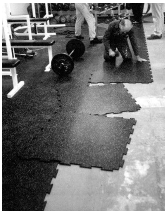
Four-Side Interlock Loose Lay Installation
